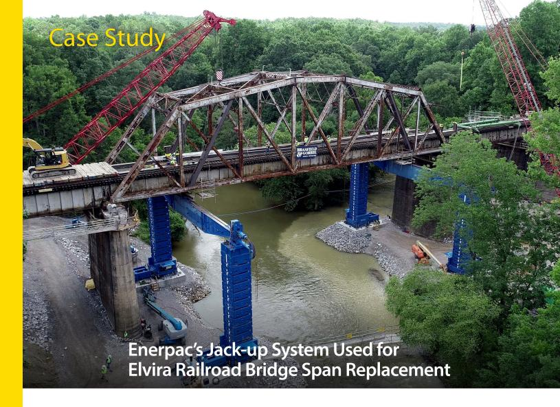
The Enerpac jack-up, a multi-point hydraulic lifting system, uses an incremental stage-lifting principle. The Elvira Railroad Bridge, built in 1906, spanned across the Cahaba River in Helena, Alabama. The old double-track open deck superstructure had reached the end of its useful life and was scheduled for replacement with a new single-track ballasted deck superstructure. Burkhalter, lifting, rigging and transport professionals, was selected to execute the replacement of Span 2 over the river.
