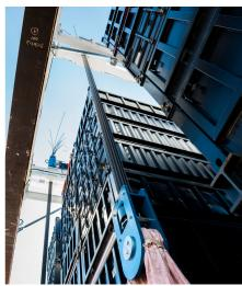
electric trolley system mounted on steel tracks and moved to a maintenance area. Installing the replacement generator is the reverse of the "Pick, Skid and Drive" process, providing the ability to complete a generator exchange within a day.
