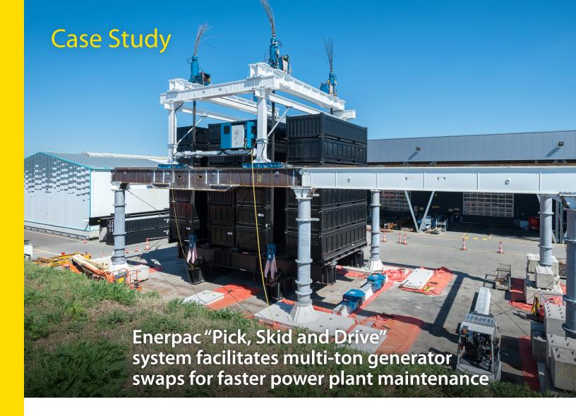
Enerpac Heavy Lifting Technology has developed a strand jack gantry system for power plant maintenance activities, allowing complete generators and turbines up to 450 tons to be swapped out within 24 hours. The Enerpac "Pick, Skid and Drive" strand jack gantry reduces maintenance time and complexity, greatly minimizing downtime disruption to power generation capacity.
